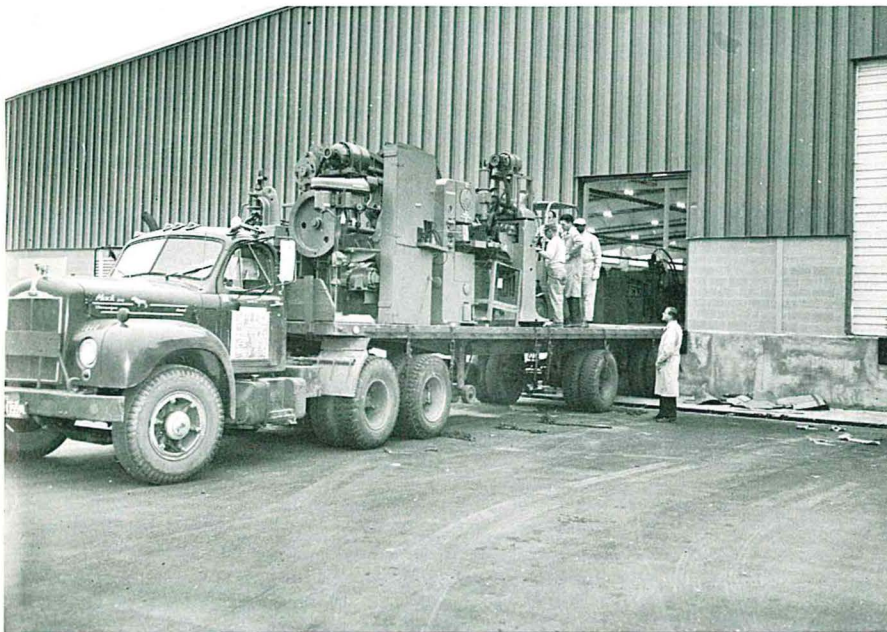
Under supervision of the Methods & Planning Department, workmen use a fork-lift truck to unload equipment brought here from the Cincinnati, Ohio, plant of Balcrank.
